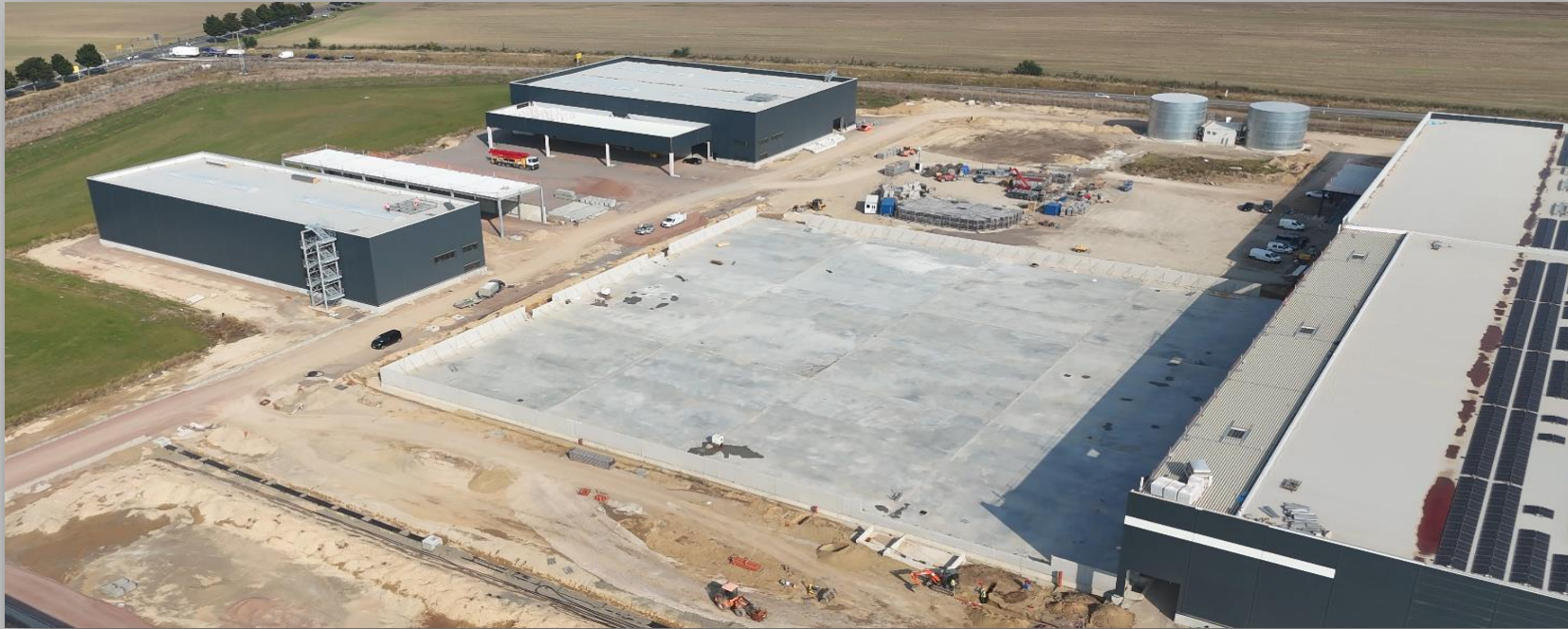
High-bay warehouse – base plate
